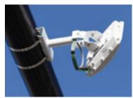
Example of a radar sensor mounted on a to what ODOT will install on existing traffic signals on OR 224/212.
